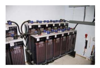
Although there are many different types of storage batteries in use, the most common and reliable by far is the deep-cycle, lead-acid battery. You may be familiar with smaller ones used in golf carts or warehouse forklift trucks. Batteries allow you to store energy when there is a surplus and hand it out when you are a bit short. So why are we using a battery bank? What other means do we have to store electricity?
